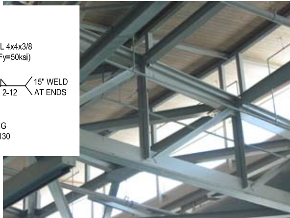
Photo & Figure 3: Adding office space atop what was previously the roof required reinforcing the existing steel roof trusses.
