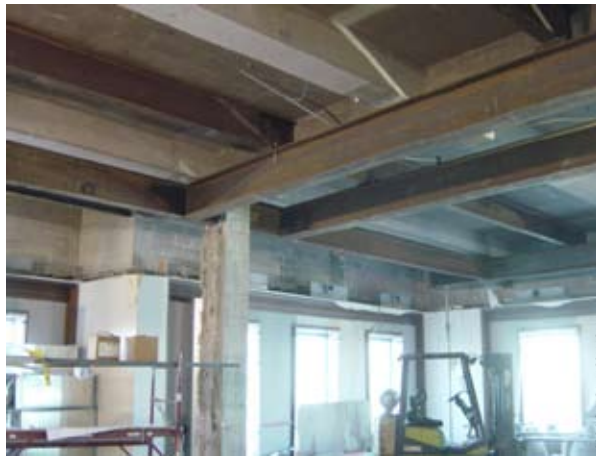
Photo 1: Adding steel grillage under the existing concrete roof structure provided additional capacity for the new floor above.
