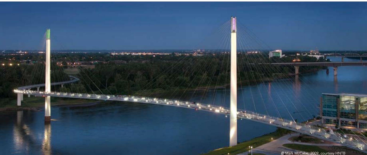
The Bob Kerrey Pedestrian Bridge provides 53 ft of clearance for Missouri River traffic and serves as a landmark for riverfront development in both Omaha, Neb., and Cedar Bluffs, Iowa.
