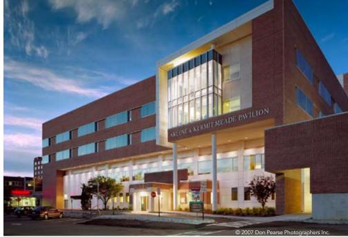
The 120,000-sq.-ft expansion of the north tower enveloped two older buildings—one a single-story steel frame building and the other a two-story concrete frame.
