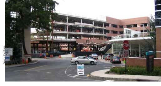
light gauge steel framing, capped by three levels of brick cladding. What is not readily apparent is that the metal panel and brick façade is actually a pre-fabricated panel system consisting of either composite aluminum panels or thin brick facing on light gauge framing supported by the main structural system. This structural system supports both the gravity and lateral loads created by the panels.
