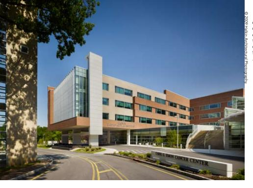
Cantilevered steel beams over the Gagnon Cardiovascular Institute's new reception and drop-off area carry column loads from the three current stories. They also have the capacity to support the addition of two more floors in the future.
