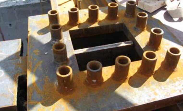
Connector plates were provided on level 16, atop the transfer truss upper chord, to receive loads for each of the concrete columns.
