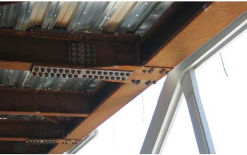
Above: Using bolted connections for the nodes of the horizontal elements in the rectangular box truss facilitated field installation.
