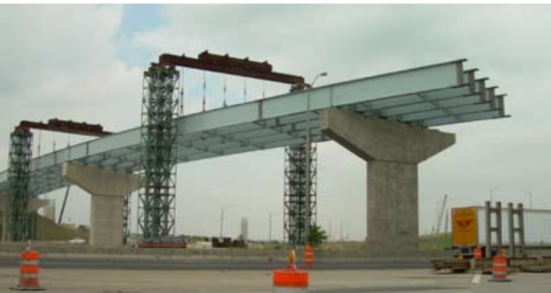
Fig 1. Typical Curve Girder During Erection
