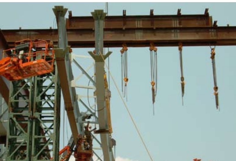
Fig 11. Connection of Adjacent Curved Girder Cross Bracing
