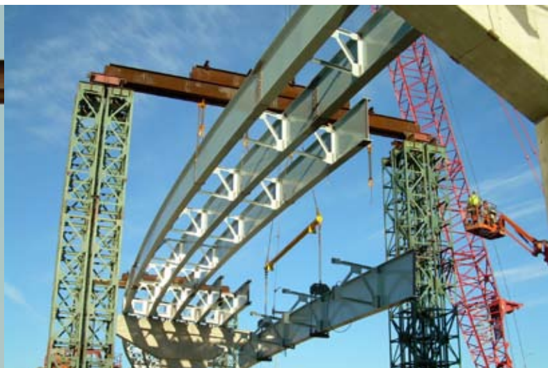
Fig 12. Typical Girder Lifts
