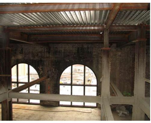
Additional steel framing facilitated the development of individual condominium units inside the old power generation station. Photo: Wexler Associates.
