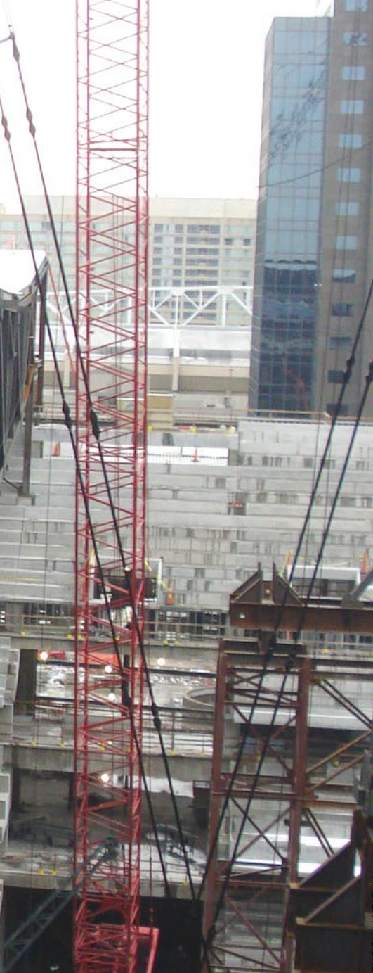
The segmentation of the primary truss top chords achieves the roof's distinctive curvature. After each half of the roof structure is independently de-centered, they will be connected with steel framing across the center bay.
