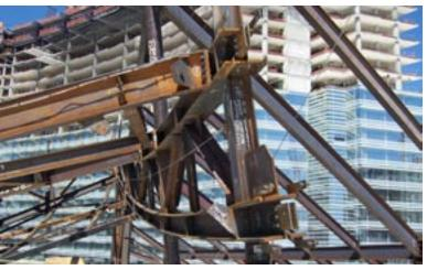
Extra tabs and attachment points had to be provided for the variety of cables that stabilized structural elements throughout the steel erection.
