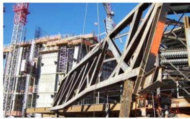
Lifting devices engineered to allow the crane to hold members at the proper skew and slope reduced the brute force required of the ironworkers in making connections.
