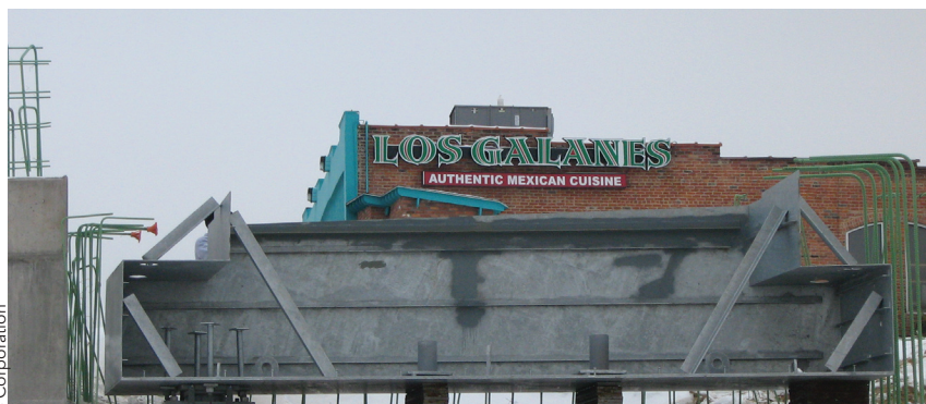
The west abutment prior to setting the tub girder. Note the non-symmetrical support system, with hold down anchorage on the left and bearing on the right.
