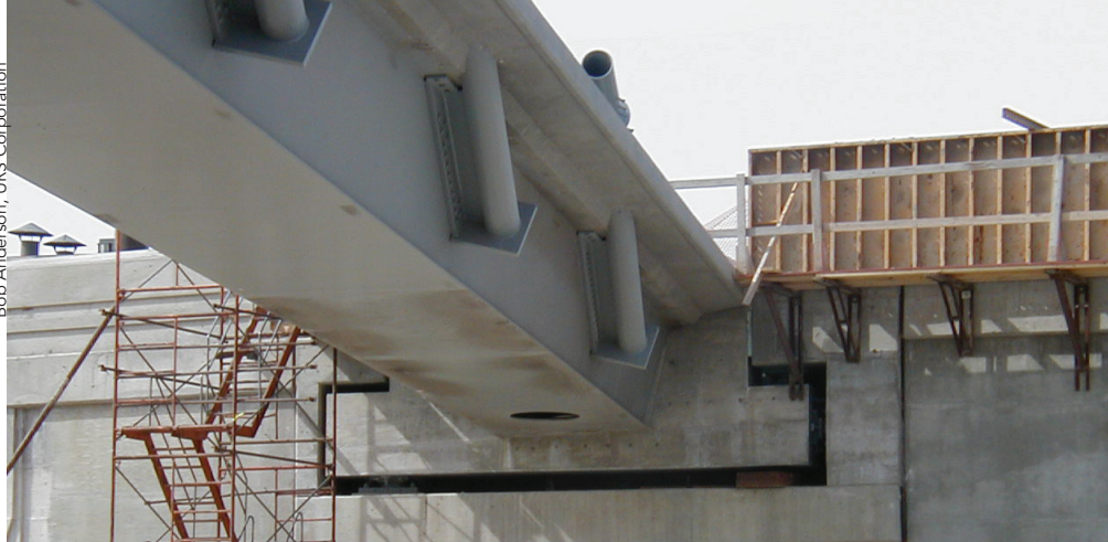
The completed west abutment.
