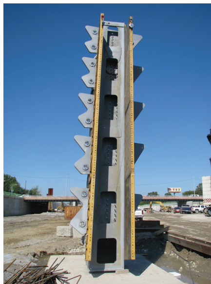
The 30-ft, 6-in.-high steel pylon stay cable housing forms the northern half of the top pylon stem, shown here prior to placement with concrete formwork panels attached. Five 2 1/2-in.-thick plates have two pinholes on one side and one pinhole on the other for connecting the clevis-type stay cable anchorages.
