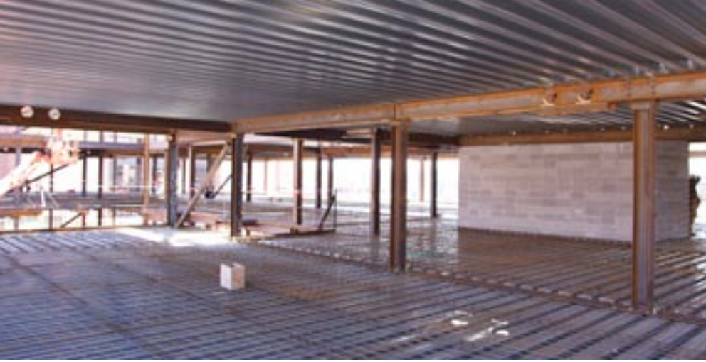
Photos this page: Versa-Floor [HR] before and after concrete
