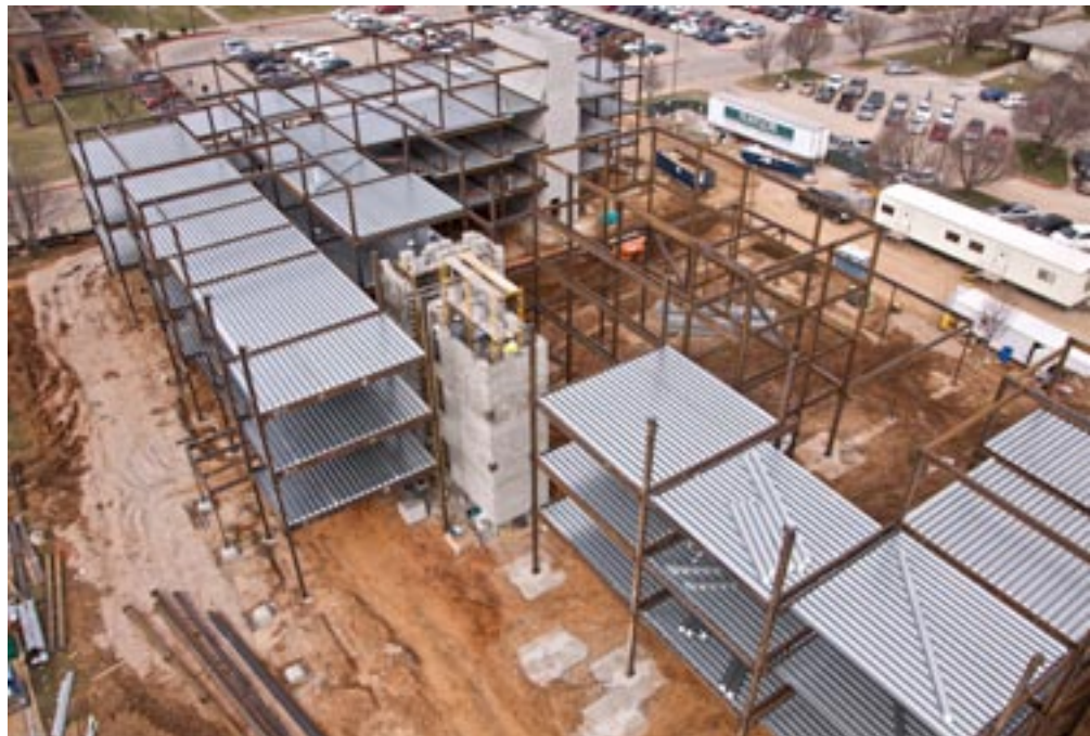
Site-fabricated Versa-Floor [HR] floor panels installed in only 18 days.
