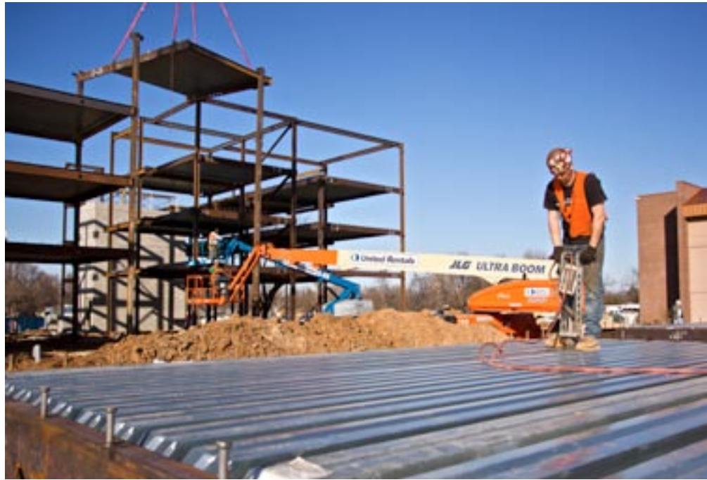
Panel fabrication and erection phases occur simultaneously.
