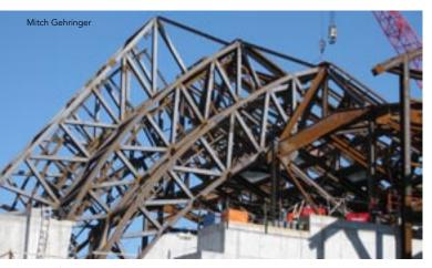
The curved organ trusses (three are visible here) echo the shape of the outer shell and form the back wall of the organ chamber. Located at the north end of the structure, they consist of eight curved vertical trusses each approximately 47 ft in height and extend from the concrete frame at Level 8 and connect to one of two trusses at the top.
