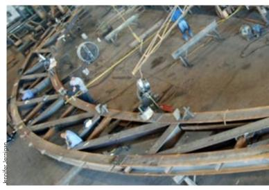
The framing for the sloped roof of the concert hall prior to its being enveloped by the curved outer shell. The concrete box in the background is the proscenium theater.
