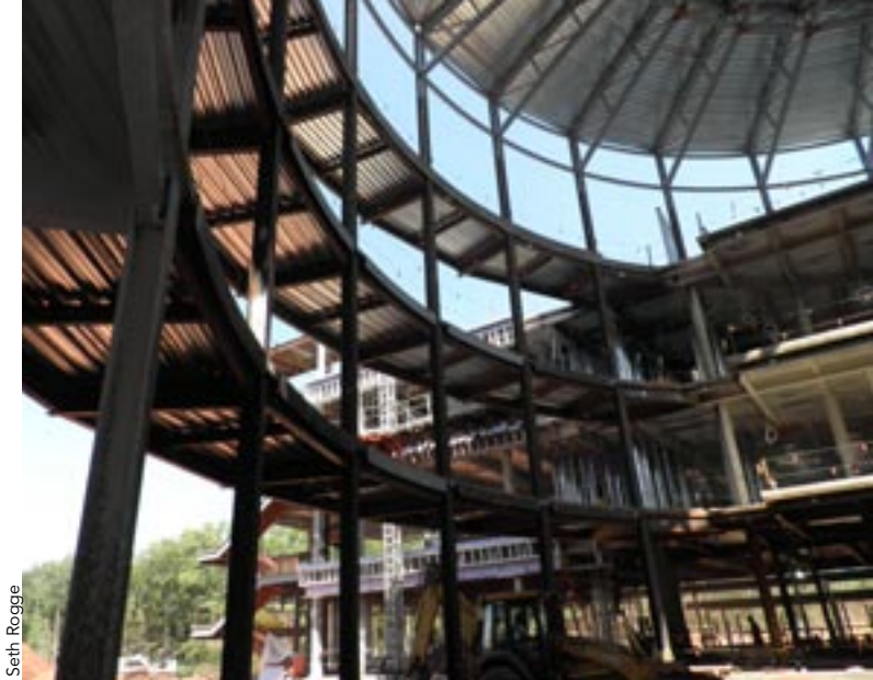
▲ The added weight of the cantilevered bridges connecting the two wings helps brace the columns supporting the dome and counterbalances the weight of the truss dome.
