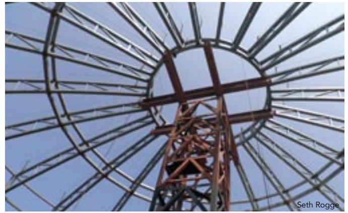
▲ Looking up at the compression rings of the dome.
