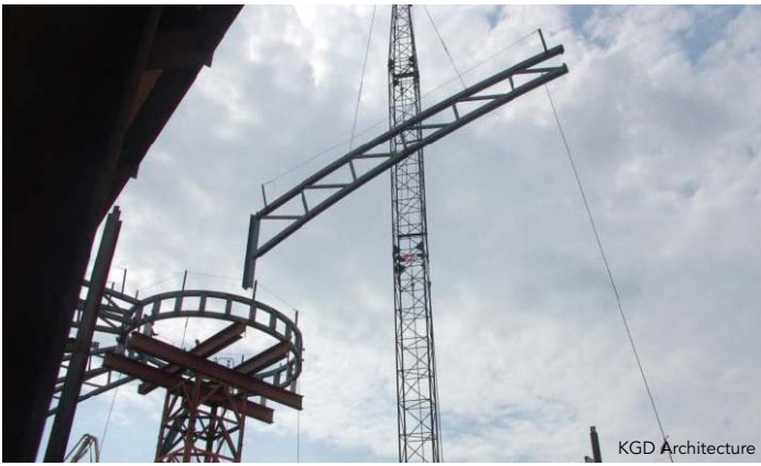
▲ One of the tapered trusses being lifted into position.
