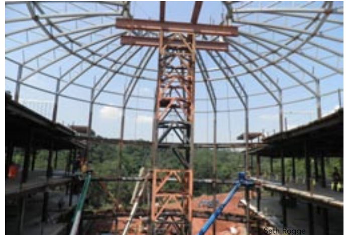
▼ Looking west from the third floor toward the dome. The vertical members at the outside end of the trusses splice directly to wide-flange columns set every 15 degrees.
