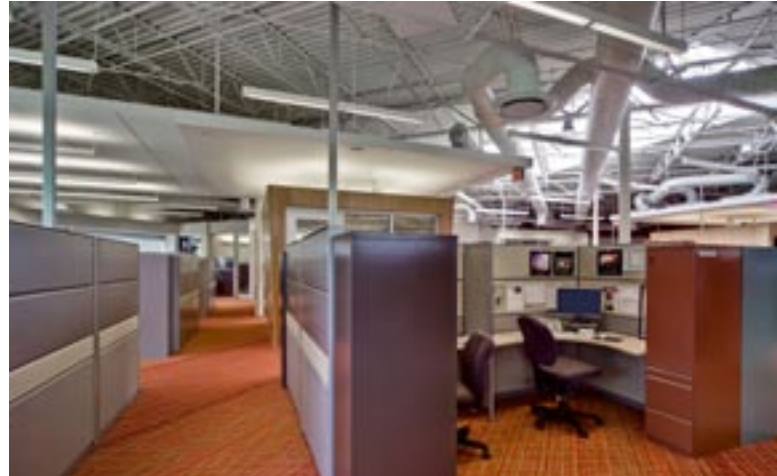
▲ Retrofitting an existing steel-framed building on the campus in the first phase of construction permitted its use while the rest of the construction continued. It also contributed to the LEED certification effort.
