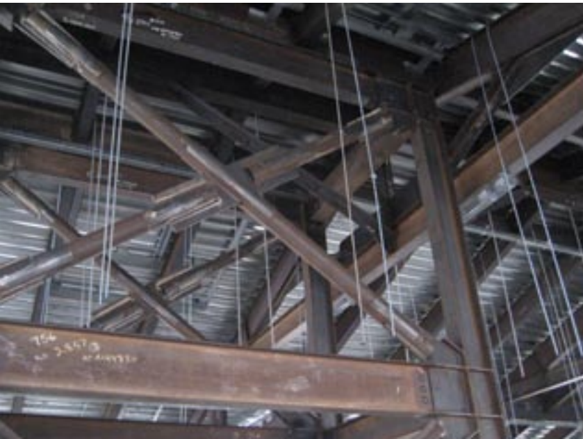
▲ As-built special concentrically braced frames. ▼ Winter construction.
