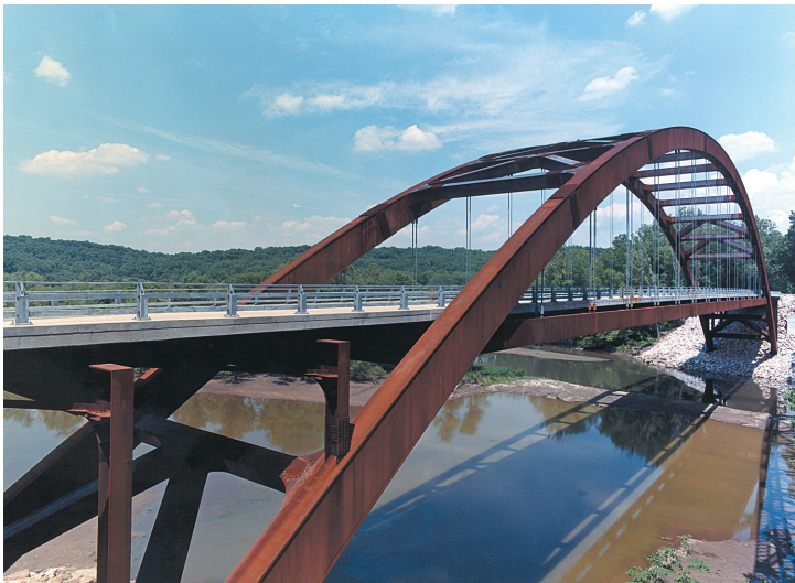
▲ 2001 Prize Bridge Award—Long Span: The Paper Mill Road Bridge in Baltimore County, Md., features a steel box arch.
