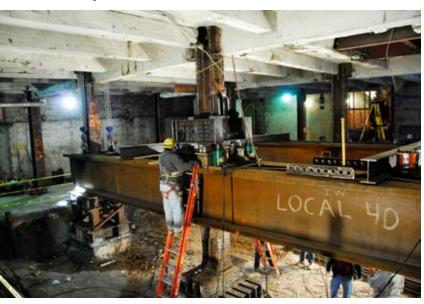
Steel bearing pedestals ensured the redistributed and transferred loads were properly induced into the outer columns and footing system.
