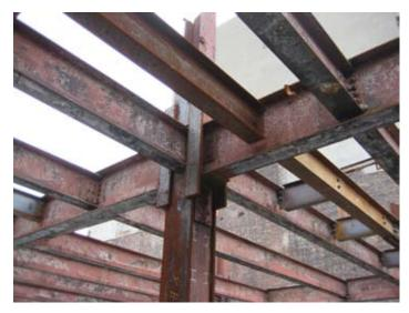
Most of the warehouse's original steel framing remained in place for the new, taller, repurposed structure. Some concrete floor slabs were removed before raising the superstructure to lighten the dead load and facilitate the foundation upgrade.
