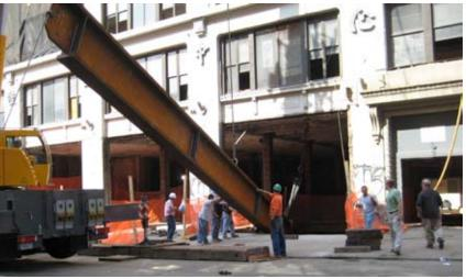
One of four 44-in.-deep, 50-ksi built-up steel plate girders with 3½-in.-thick flanges being lowered into the basement. The girders transferred column loads of as much as 900 kips and facilitated a foundation replacement under existing columns.
