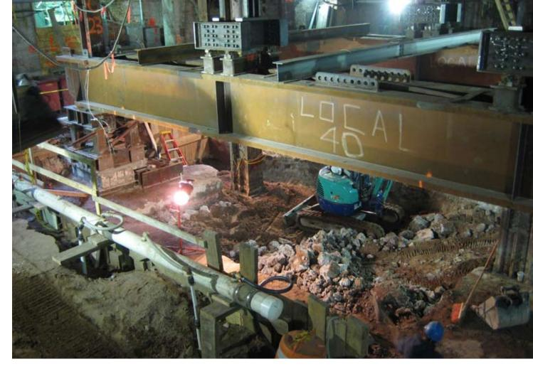
After the jacking process relieved the load on the interior columns, the existing foundation in that area was demolished and replaced with a larger, deeper mat foundation.
