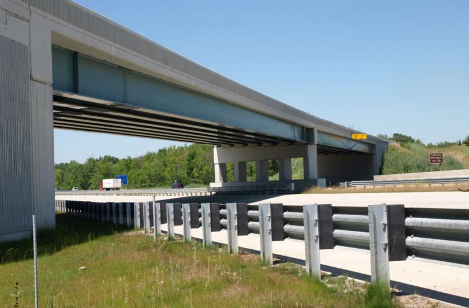
▲ The completed structure showing the new span to the left of the new median pier.
