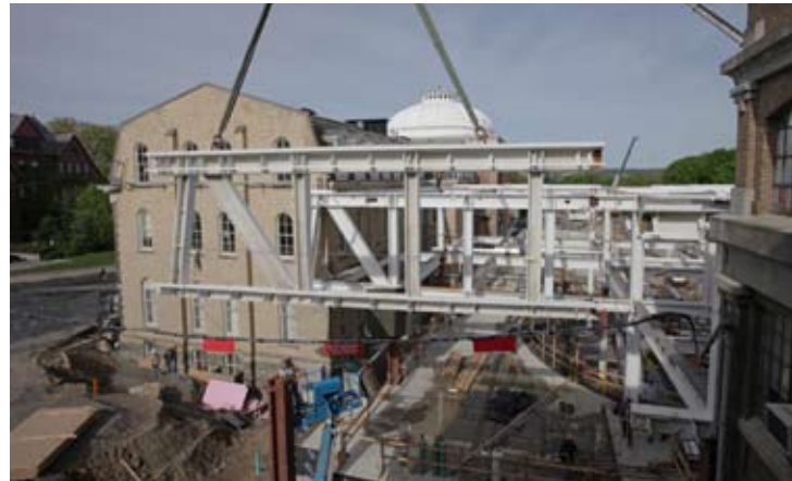
▶ Fabricated structural steel truss sections trucked to the site on a closely coordinated schedule kept the main framing erection to just four weeks.
