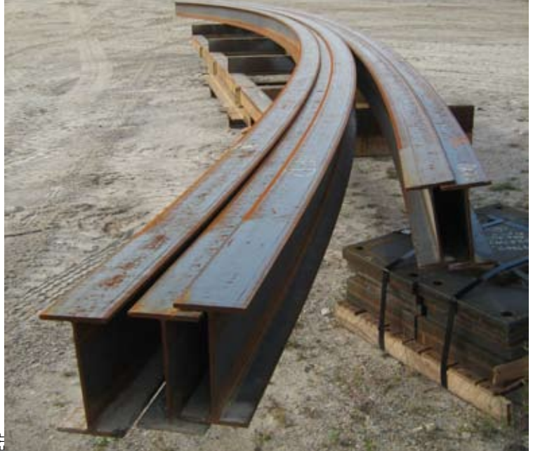
▲ Careful planning reduced the number of horizontally curved beams in the office wing to a minimum.
