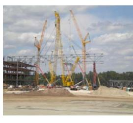
▲ The initial sway brace assembly being hoisted into place.
