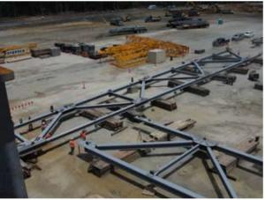
▲ The 610-ft-long trusses were assembled on the ground in two sections.
