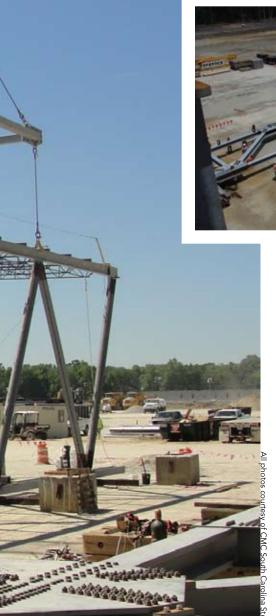
A Sway trusses 100 ft long and 25 ft apart provide the bracing for the main trusses and were also assembled on the ground before being hoisted into place.
