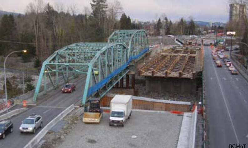
▲ New steel girders being launched from the Capilano River's east bank, over the river pier and closing in on west abutment.
