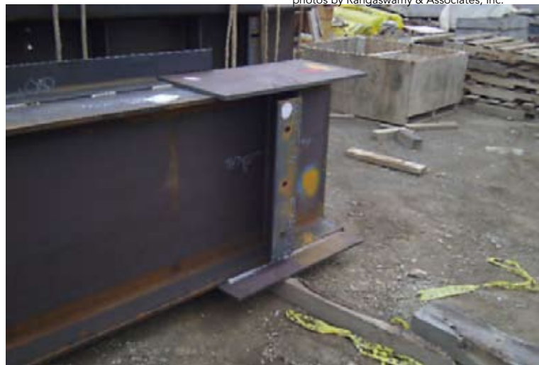
▲ Beam end of the connection.
