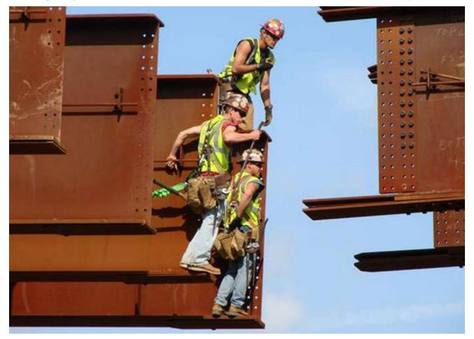
A Ironworkers prepare to field splice the plate girders on the West Virgina approach to the Blennerhassett Island Bridge, which used high-strength, high-performance 70 ksi weathering steel for maximum durability and improved ductility.
