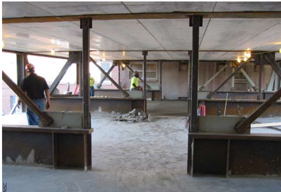
▲ Exterior elevation of the addition. The cantilevered study lounges are on the right. ▼ Notch in upturned girder at the corridor.
