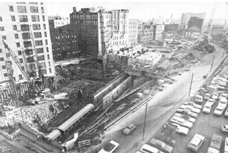
▲ Construction of the original foundation.
