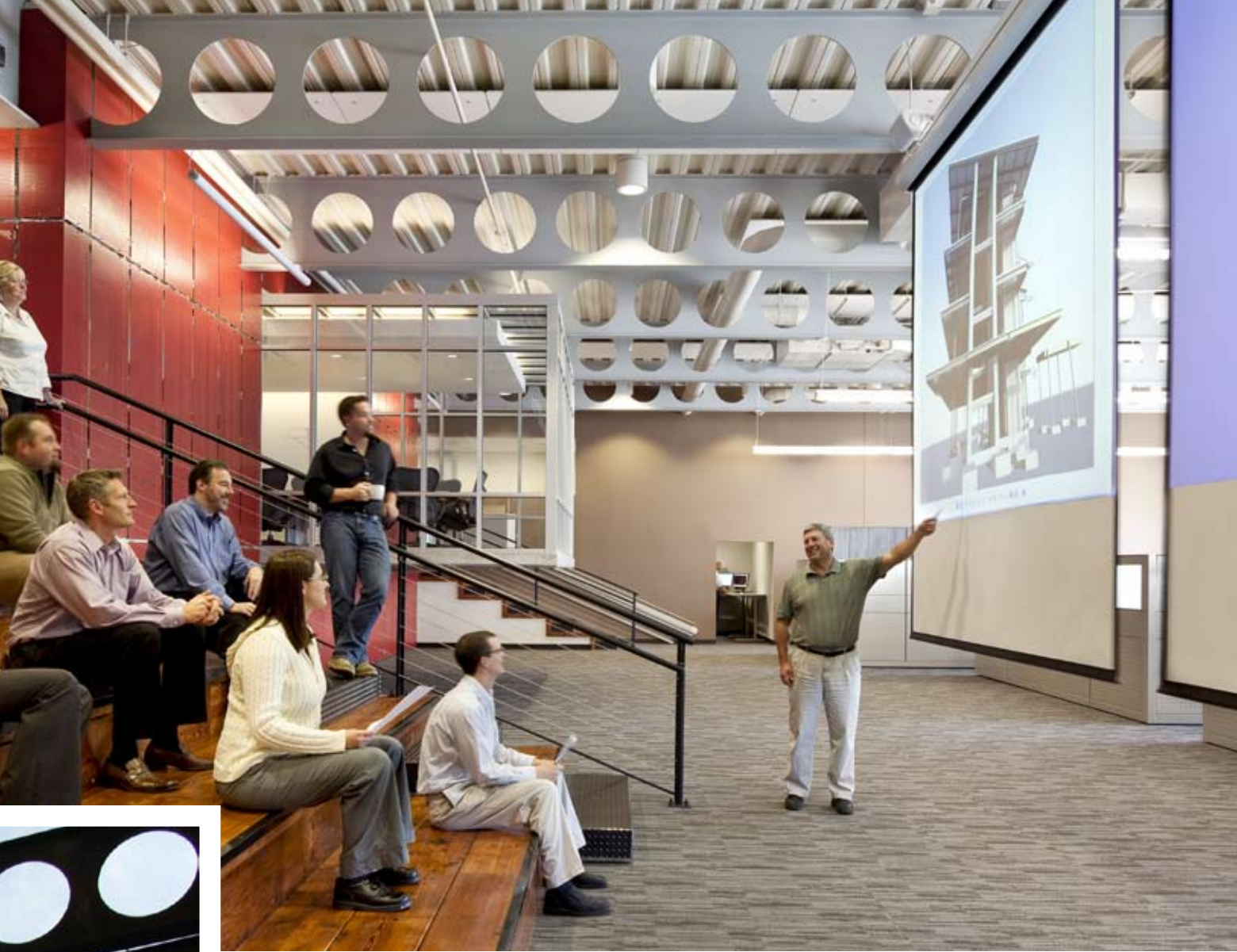
▲ PCS's finished space showcases exposed cellular structural steel framing in the conference room and amphitheater areas.
