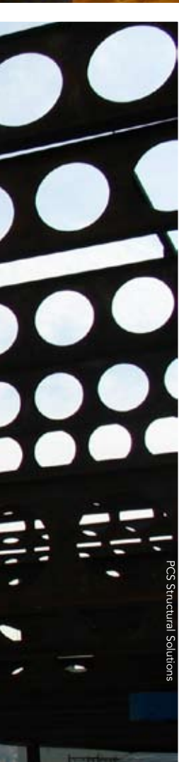
▲ PCS's finished space showcases exposed cellular structural steel framing in the conference room and amphitheater areas.
