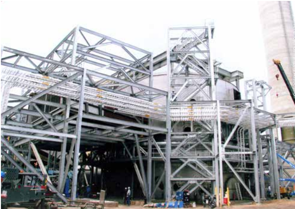
▲ While power plants have long been built with traditional steel frames (above), there has been a recent increase in modular framing design for these facilities.
