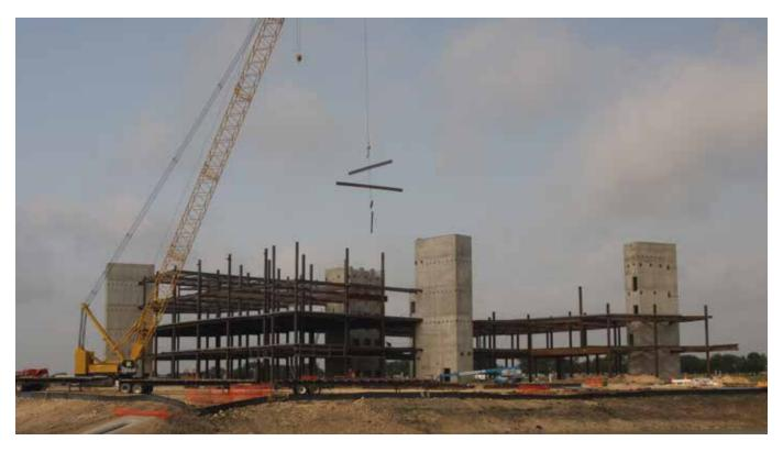
Texas Health Harris Methodist Hospital Alliance, an IPD steel project, was detailed and fabricated by Alpha/SteelFab after they assisted in converting the design from the original concrete concept.
