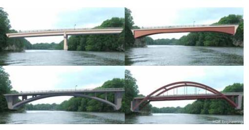
▲ The four bridge alternatives that were considered. Clockwise from upper-left: a prestressed concrete girder, a haunched steel girder, a partial through steel arch (the selected design) and a concrete deck arch.
