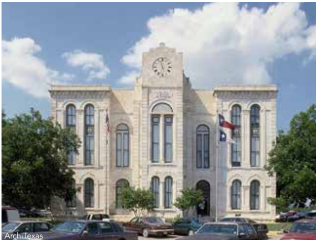
▲ The Bosque County Courthouse, prior to restoration.
