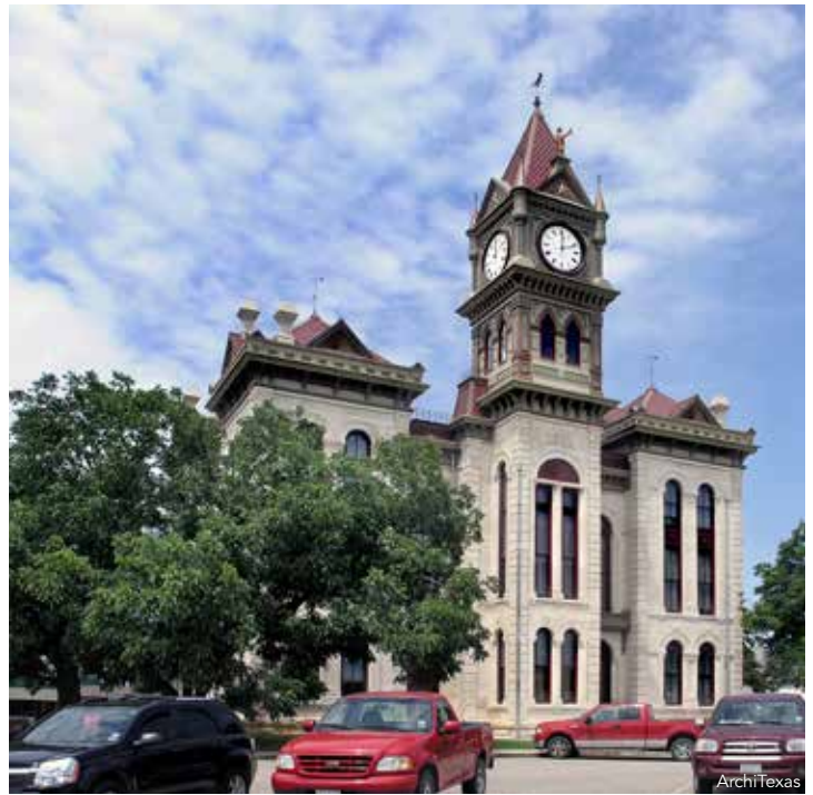
▲ Completed restoration of the courthouse.
