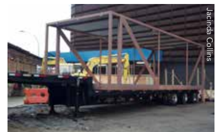
▲ One of the structural modules for B2.
