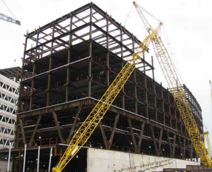
▲ The main office building uses 23,000 tons of structural steel.
