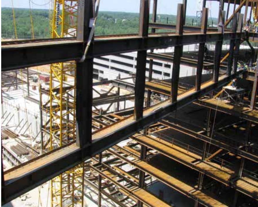
▲ Lifting one of the Vierendeel trusses.
