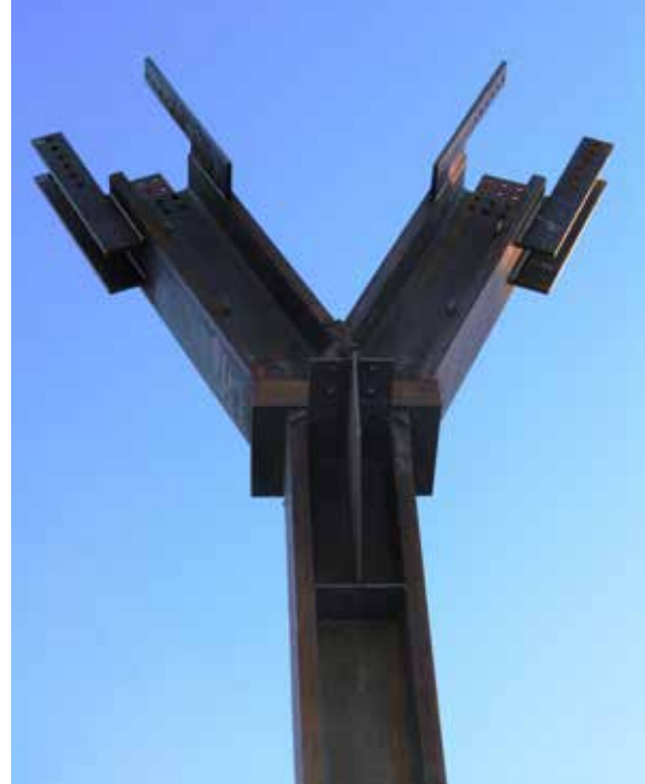
▲ A base for one of the V columns.
