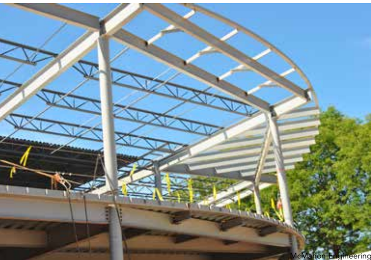
▲ The steel roof framing system consists of a metal deck supported by steel joists and steel beams. This system allowed for a large curved façade and accompanying 5-ft overhang to be relatively simple and repeating.
