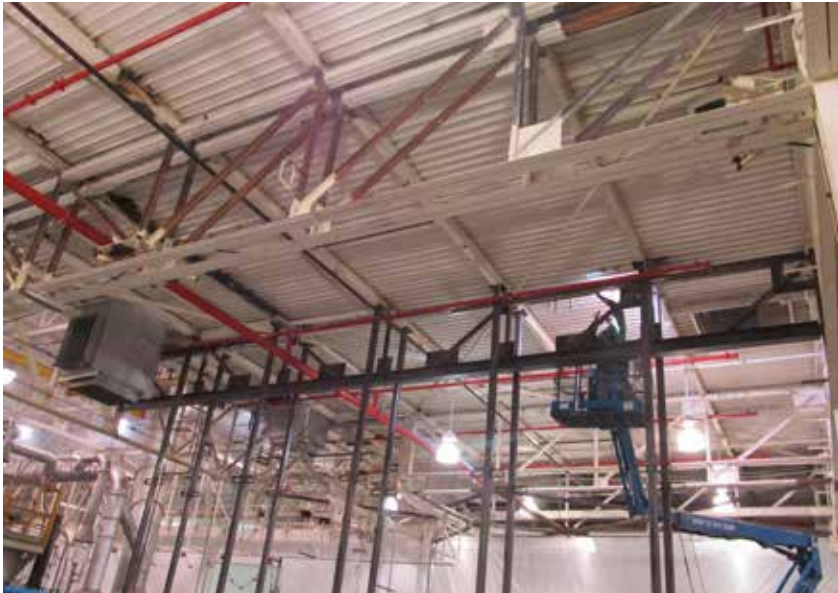
◀ Installation of the new bottom chord.
