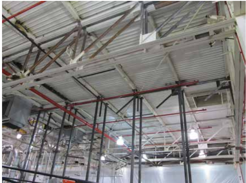
▲ Truss with the bottom chord removed.
