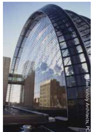
➤ The Kimmel Center for the Performing Arts features a curved steel barrel vault that measures 350 ft by 174 ft in plan.
