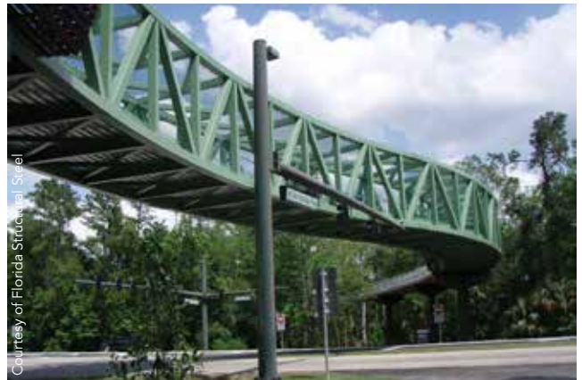
▲ The Seminole County pedestrian bridge.
