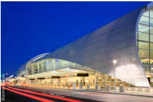
▲ The expansion of the Mineta San Jose International Airport Terminal B and Concourse used 420 tons of curved steel.
