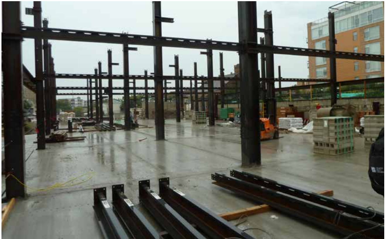
▲ Steel framing for the first floor, including the D-beams.
