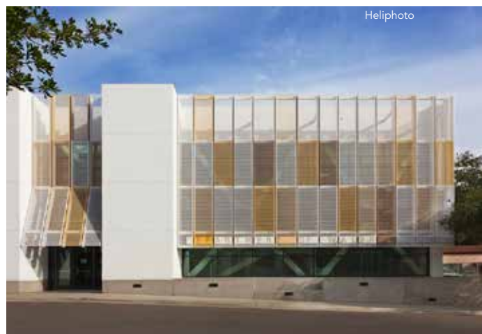
▼ The perforated metal panel system of the west elevation.
