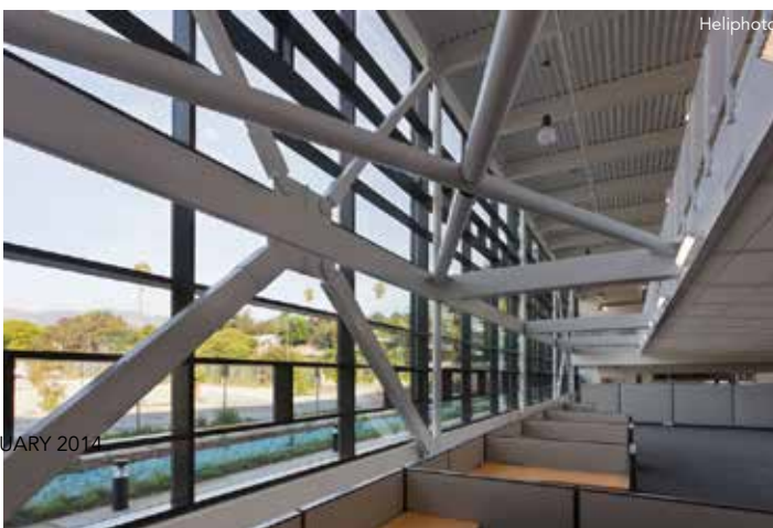
▼ The horizontal truss at the second floor of the north elevation.
