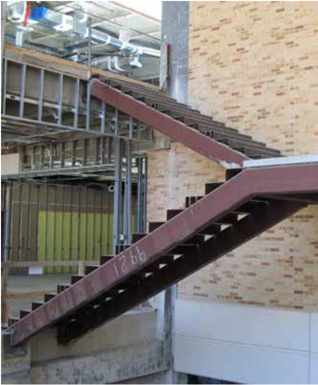
▲ The interior scissor stair under construction...
