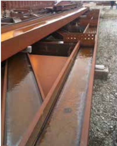
▲ Fabricated steel was exposed to the elements for four years before reuse. ▼ The completed structural frame.
