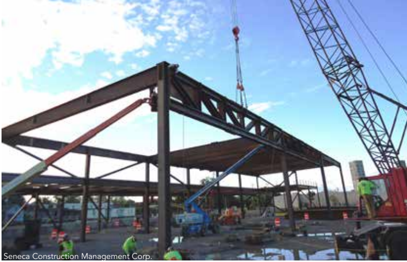
◀ Erection of a reused steel truss.
