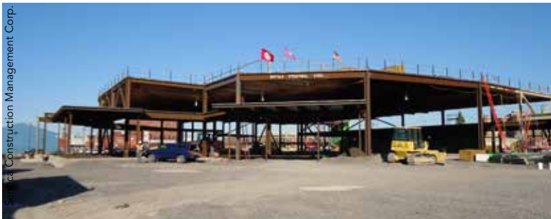
▲ Fabricated steel was exposed to the elements for four years before reuse. ▼ The completed structural frame.
