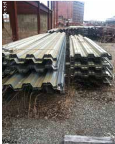
▲ The project team was concerned about potential corrosion caused by trapped moisture in the nested sheets of composite metal deck.
