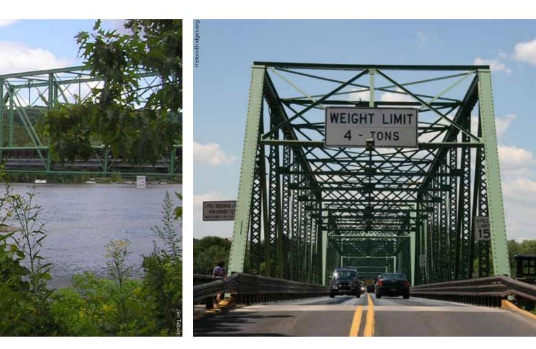
The New Hope-Lambertville Bridge opened in 1904 and currently carries 14,000 vehicles across the Delaware River daily. Each of the bridge's six spans measures 171 ft, and the total length is about 1,050 ft.Vertical truss members measure 27 ft in height, and abutments date back to the original 1814 bridge.
