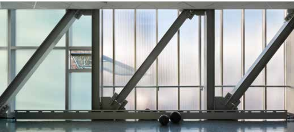
▼ The framing includes trusses of 110 ft and 120 ft long, both 13 ft tall.
