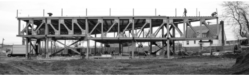
▼ The framing includes trusses of 110 ft and 120 ft long, both 13 ft tall.
