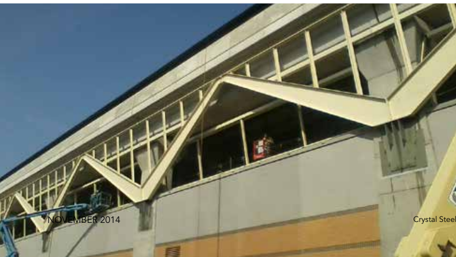
▲ Framing for a window in the Wiehle-Reston East station canopy. ▼ Steel "V's" at the McLean station.
