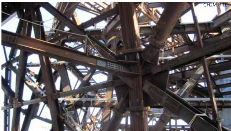
▲ ▼ A shared node with a 19.7-in. × 23.6-in. laminate diagrid member.
