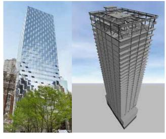
built up with 2-in. plates across the flanges, and W14×605s were used as the outriggers at the sixth and roof levels, respectively.
