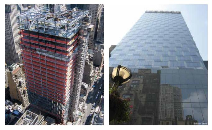
Framing for the 520-ft-tall International Gem Tower was erected in two phases, the first of which included steel for two of the belowgrade levels and the ground floor; the second phase consisted of superstructure erection.
