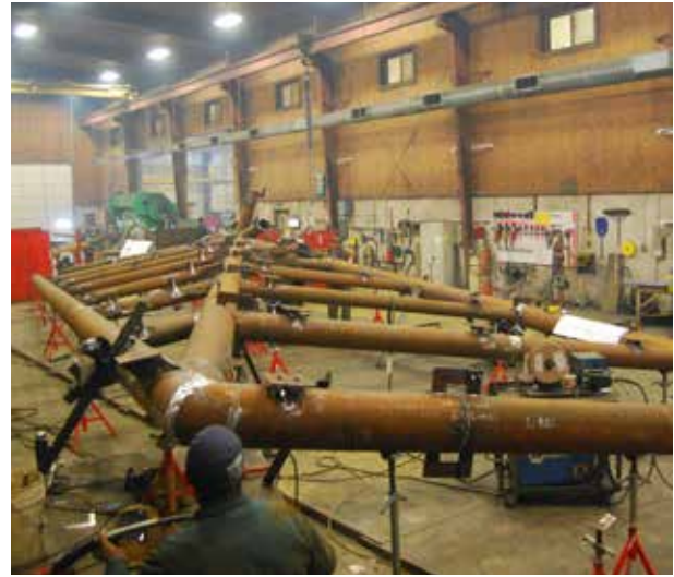
▲ The waterfall itself was made and erected to AESS standards and cleaned to the requirements of the SSPC-SP 6/NACE No. 3, Commercial Blast Cleaning standard; two coats of Tnemec Paint were applied.
