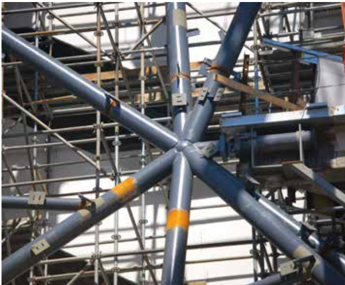
▲ One of the complex nodes of the waterfall. ▼ Twelve connection points were used to attach the waterfall frame to the building structure.
