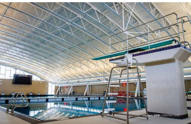
tilated pool space, they did not have as much corrosion as the roof steel. Therefore, they did not require any additional reinforcing as they already had enough capacity for the new loads.
