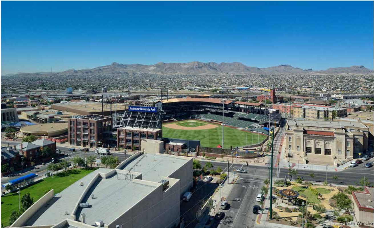
▲ The tight site required four levels (two levels of suites), rather than the two or three seating levels typical of most Triple-A ballparks. To maximize suite space, the upper suite levels are hung from the roof structure rather than posting down to the level below.
