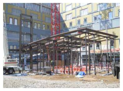
tional stone, which let the engineers design the steel support structure for higher allowable deflections than traditional stone would have allowed.
