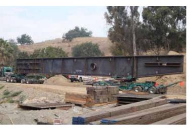
The long cantilevers are supported by a combination of two-story Vierendeel trusses and heavy steel plate girders at the roof. The heaviest steel plate girder is 9 ft deep, with a weight of approximately 82.5 tons.
