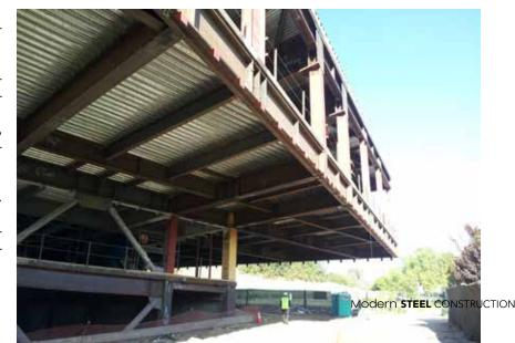
Built-up steel plate girders are located at the roof level, where larger back spans are able to counterbalance the deflection at the cantilevered building corner.
