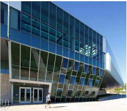
The facility features several substantial cantilevered floor areas, the longest of which extends nearly 60 ft.
